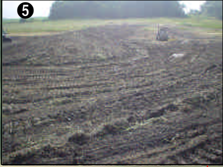
Completed Embankment and Emergency Spillway
