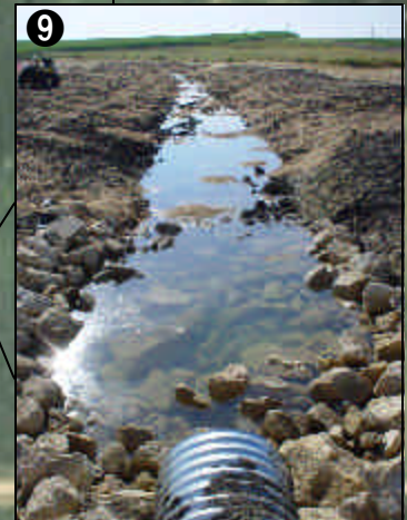
Looking East: Main Tile Outlet Pipe and Ditch
