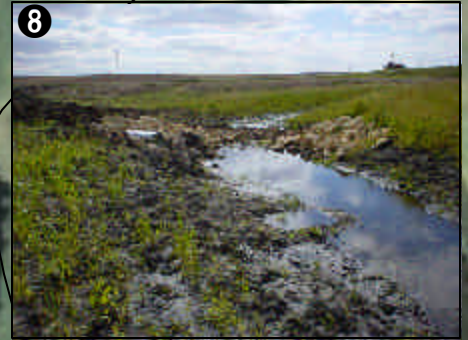
Branch #80 Outlet Structure
