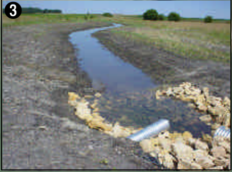
Looking North: Basin #2 Water Control Structure and Tile Reroute Outlets
