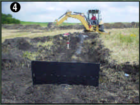
Installing Water Control Structure for Basin #2
