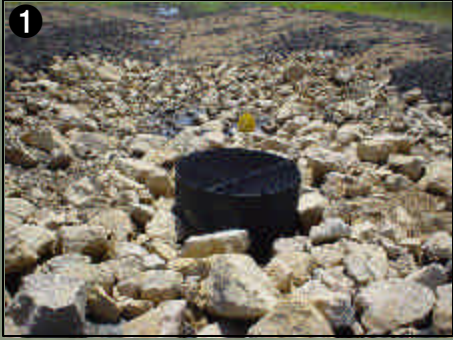
Main Water Control Structure
